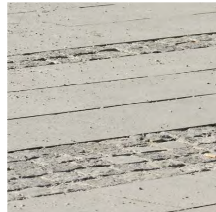
Concrete block and stone setts
